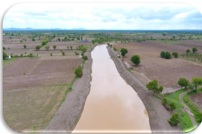
Water stored in De-silting, deepening & widening of Nalla and Ground water table increased
