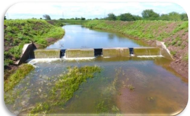
Water stored in Cement Nala Bunds and de-silting, Deepening & Widening of Nalla
